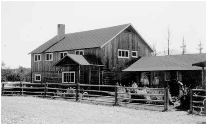
Rebuilt lodge, after the fire
