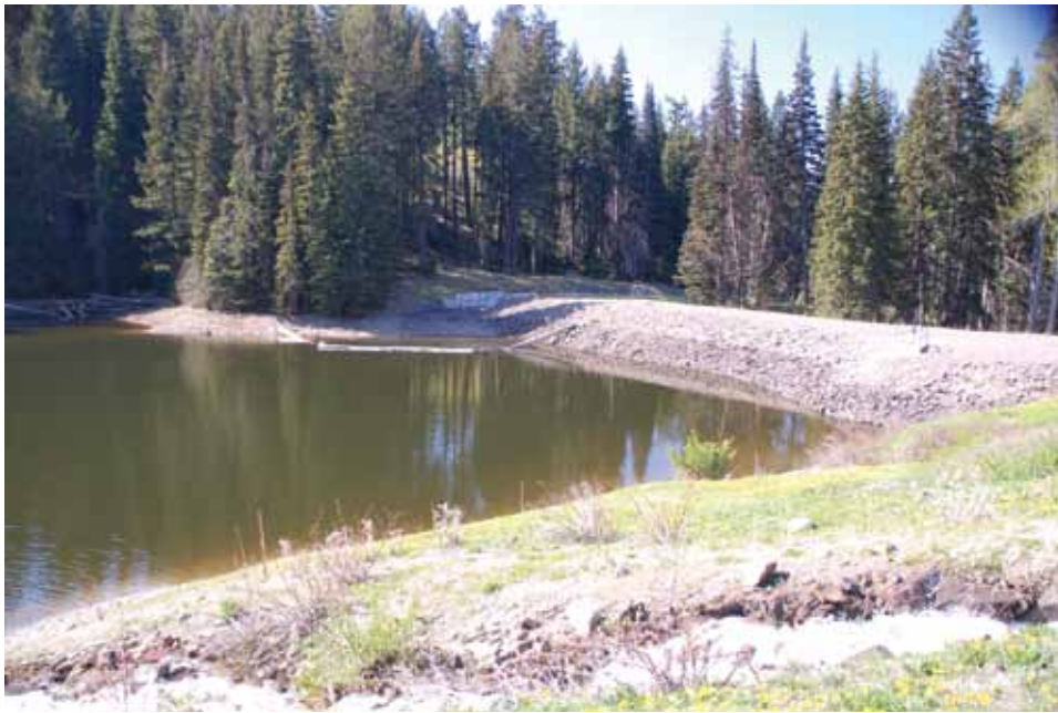
View of the dam
