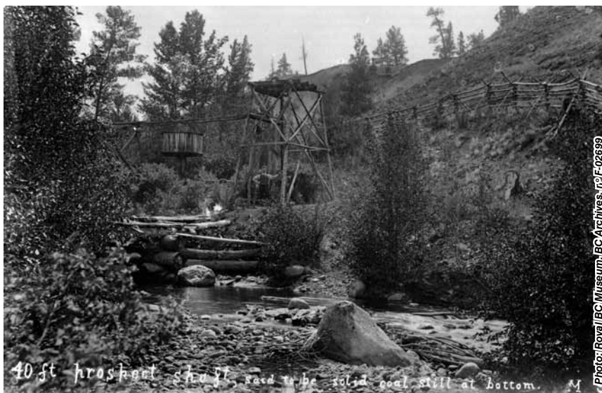
40 foot prospect shaft, Hat Creek coal outcrop, 1910.
