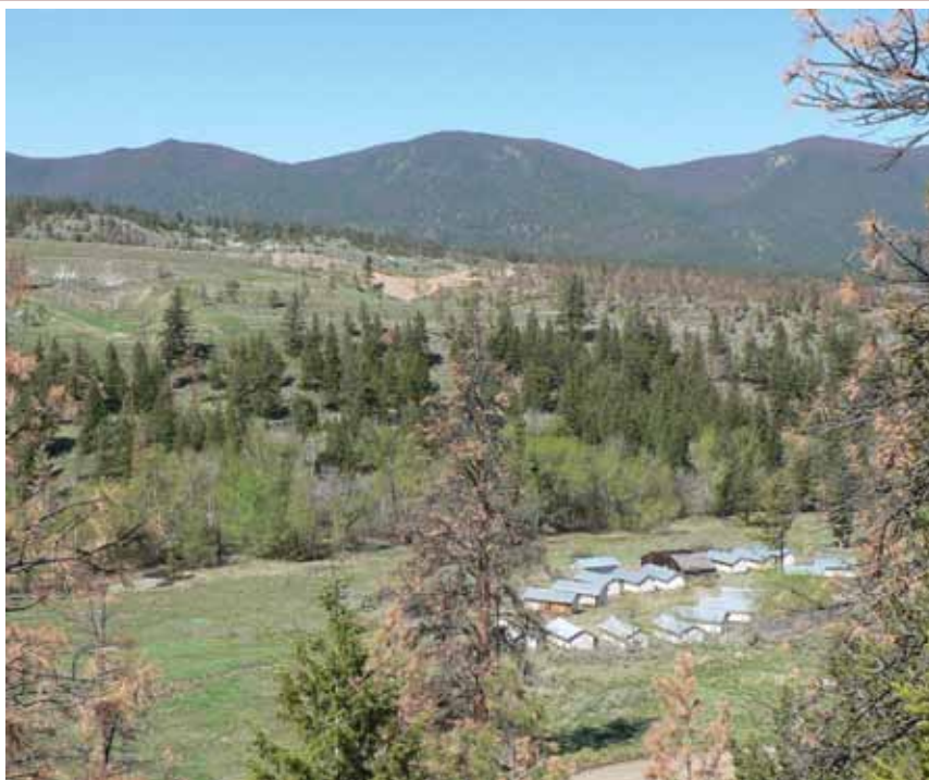
The BC Hydro compound lies below the excavation site.
