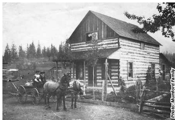
Grinder's Mountain House
