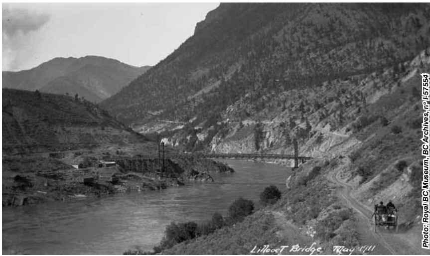
Looking up river at the Lillooet Bridge, 1911
