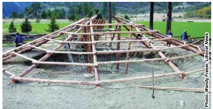
Construction of Pit House, 2006
